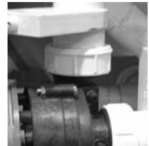
Slice Valve and Pump Union
